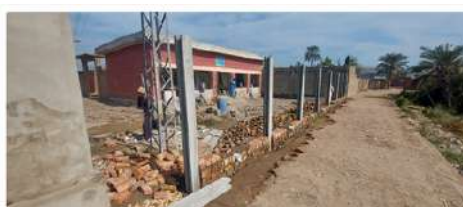
Boundary wall construction
